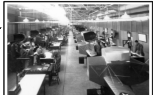
Chanute Field, 1943 Rows of Link trainers fill this classroom. These trainers were used to teach both Link trainer operators and maintenance technicians.
